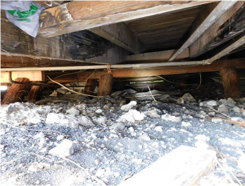
Photo 9, Crawlspace, toppled foundation piers.
